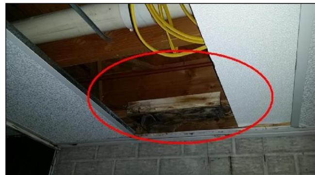
There is water damage present on the floor structure and/or sub-floor. Significant damage or weakening has occurred. Recommend evaluation and repair by a qualified contractor.
