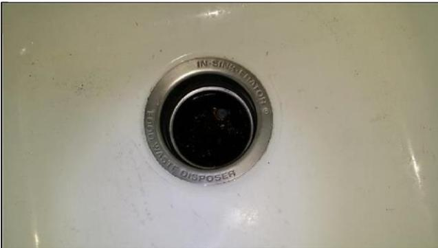
The rubber boot is damaged and should be replaced for safety and proper function. Recommend evaluation and repair by a qualified contractor.
