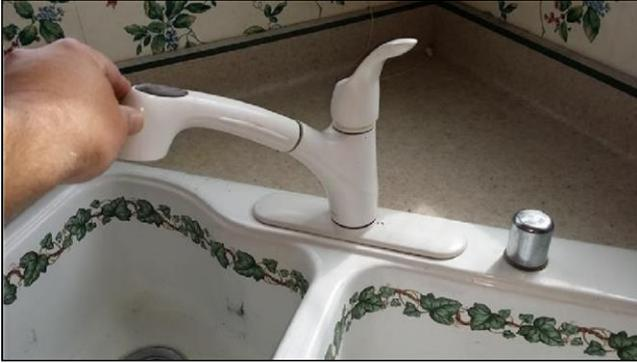
One or more faucets handles are loose and/or damaged. One or more faucet spouts are tight moving side to side. This could be from improper installation and/or some kind of damage. Recommend evaluation and repair by a qualified contractor.
