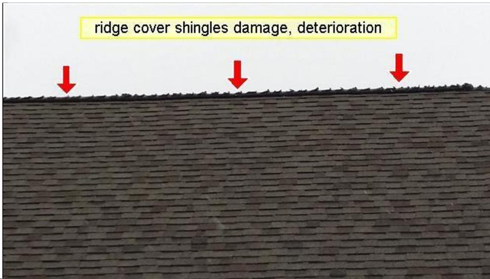
One or more areas have significant wear, deterioration, and damage, exposed felt, exposed nail heads, lifting or granular loss. One or more areas are lifted, missing or damaged. The cause is not determined. Recommend evaluation and repair by a qualified contractor.
