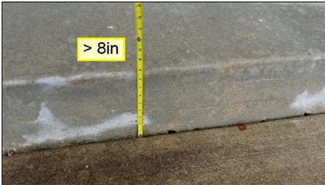
There is walk settlement that is causing the step height to be greater than 8in. Recommend evaluation and repair by a qualified contractor. Reconstruction may be necessary.
