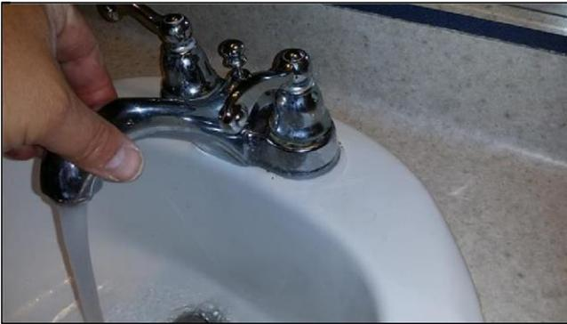
One or more faucets are loose and need to be properly tightened (upstairs hall). Recommend evaluation and repair by a qualified contractor.
