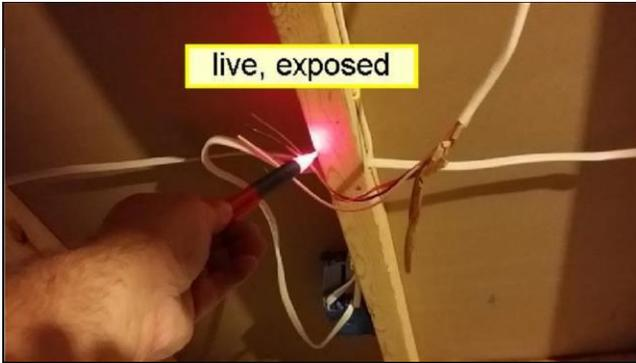
There are one or more exposed cable/conduit wires present. Recommend evaluation and repair by a qualified contractor.
