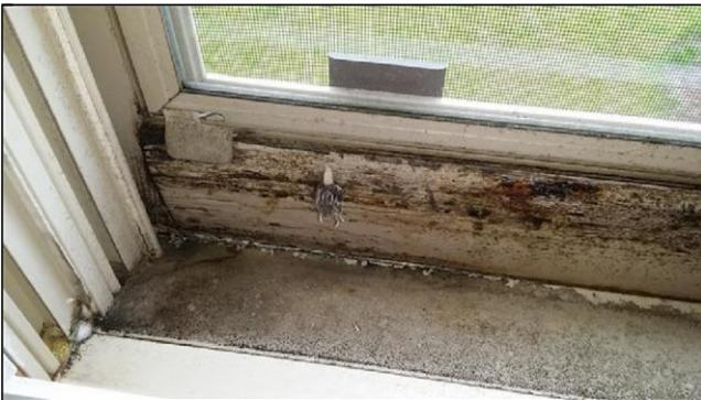
One or more storm windows are broken, cracked, damaged or have significant deterioration. Recommend evaluation and repair by a qualified contractor.
