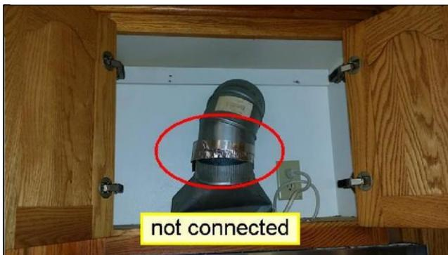
The exhaust duct work is damaged, not connected or not connected properly. Recommend evaluation and repair by a qualified contractor.
