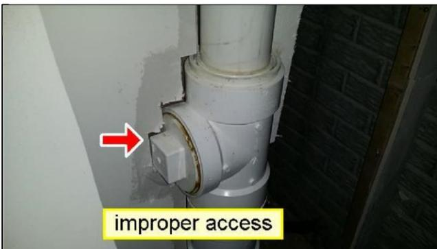
One or more clean out covers are not accessible. Remove the obstruction or move the cleanout. Recommend evaluation and repair by a qualified contractor.
